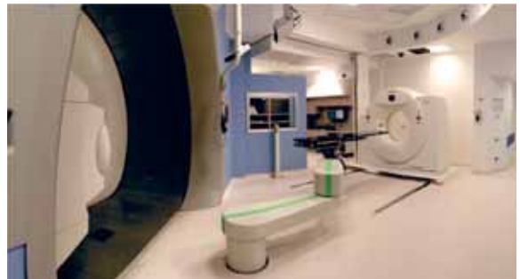
Figure 10: The ‘on-rail’ CT available in one of the treatment rooms in Trento.
