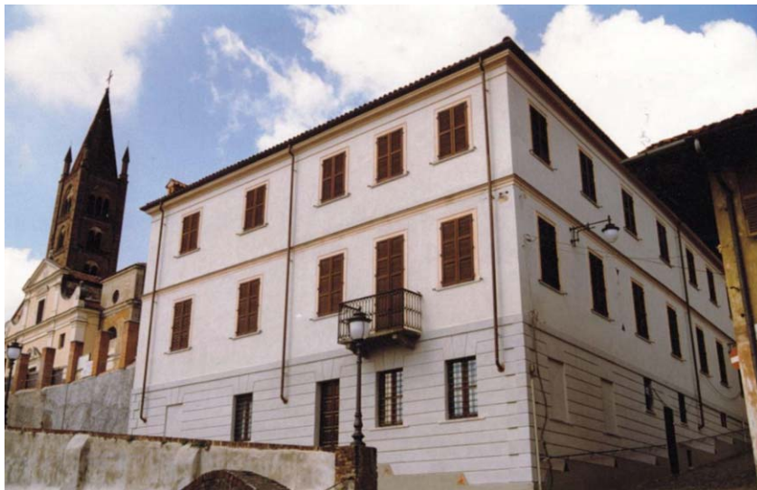
Fig. 2. “Casa Capello” in Rivoli. On the background the bell tower of the Collegiata, on the foreground the breast wall that collapsed during the restoration works.
