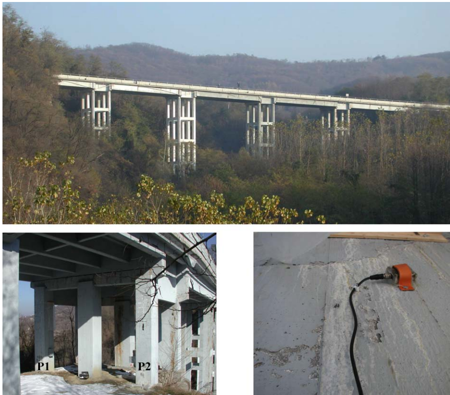
Fig. 10. The viaduct and the monitored pilasters P_1 and P_2 with the applied sensor.
