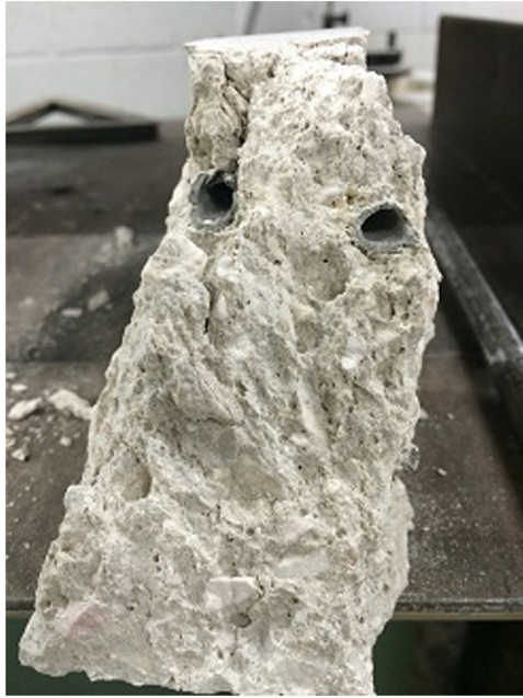
Figure 1. Fragment of the cubic specimen with horizontally oriented hollow tubes after failure in compression: two fractured hollow tubes are visible at the top of the fragment and the good adhesion between the tubes and the cementitious matrix can be noted.
