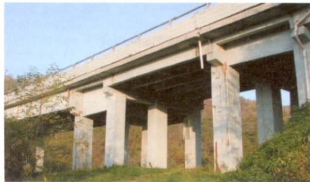
Fig. 2 : The monitored viaduct
