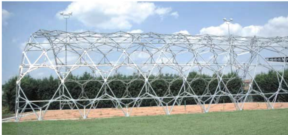
Fig. 30. Tennis court cover Racconigi (Courtesy G.T.C.A. Srl Grid Structures).
